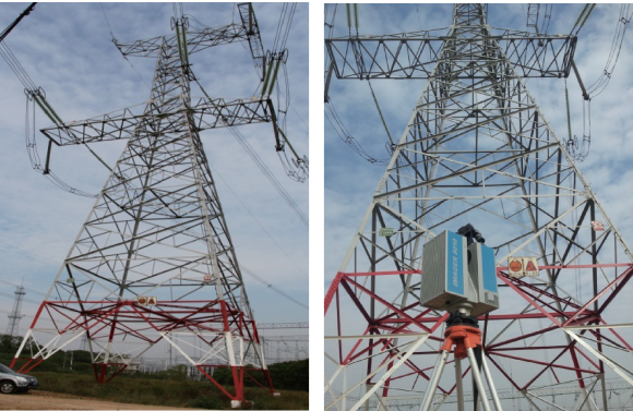
(a) 被测杆塔图片 (a) Picture of tested tower (b) 地面激光雷达采集点云 (b) Point cloud acquisition by terrestrial 3D lidar
