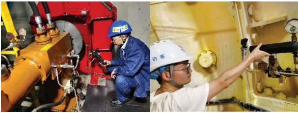
图7 灯泡头(左)与灯泡体(右)金属扫膛故障实验图 Fig. 7 The test diagram of the metal sweeping failure of the bulb head (left) and the bulb body (right)
