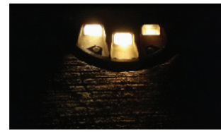
(a) 跑道边灯 (a) Runway side lights
