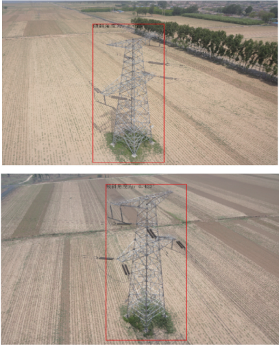
(b) 吕梁220 kV文汾线75#3个拍摄方向的检测效果 (b) Lvliang 220 kV Wenfen Line 75# inspection effect picture of three shooting directions
